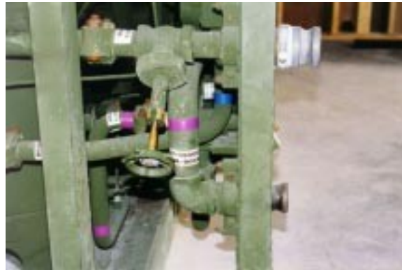
Figure 33. VENT VESSELS Gate Valve.
