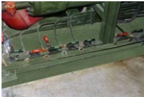
Figure 32. Drain Valves.
