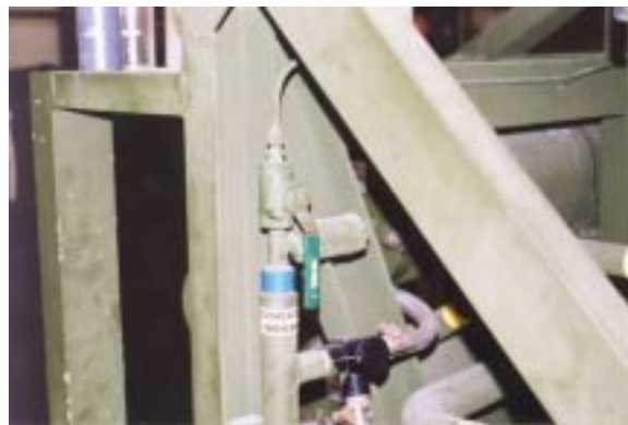
Figure 34. VENT PRODUCT WATER Valve.
