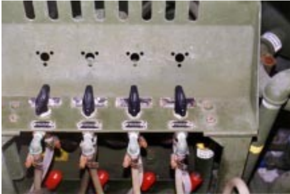
Figure 37. Chemical Feed Run/Prime Values in PRIME Position.
