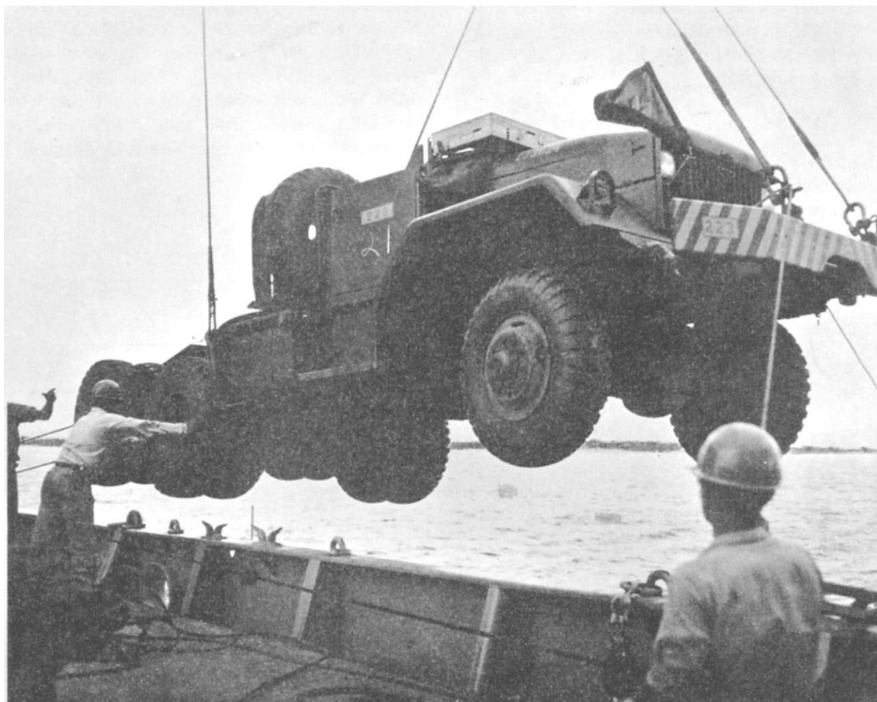
Figure 9-21.—Bridle legs may be attached to hoisting padeyes of unloaded military vehicles.
