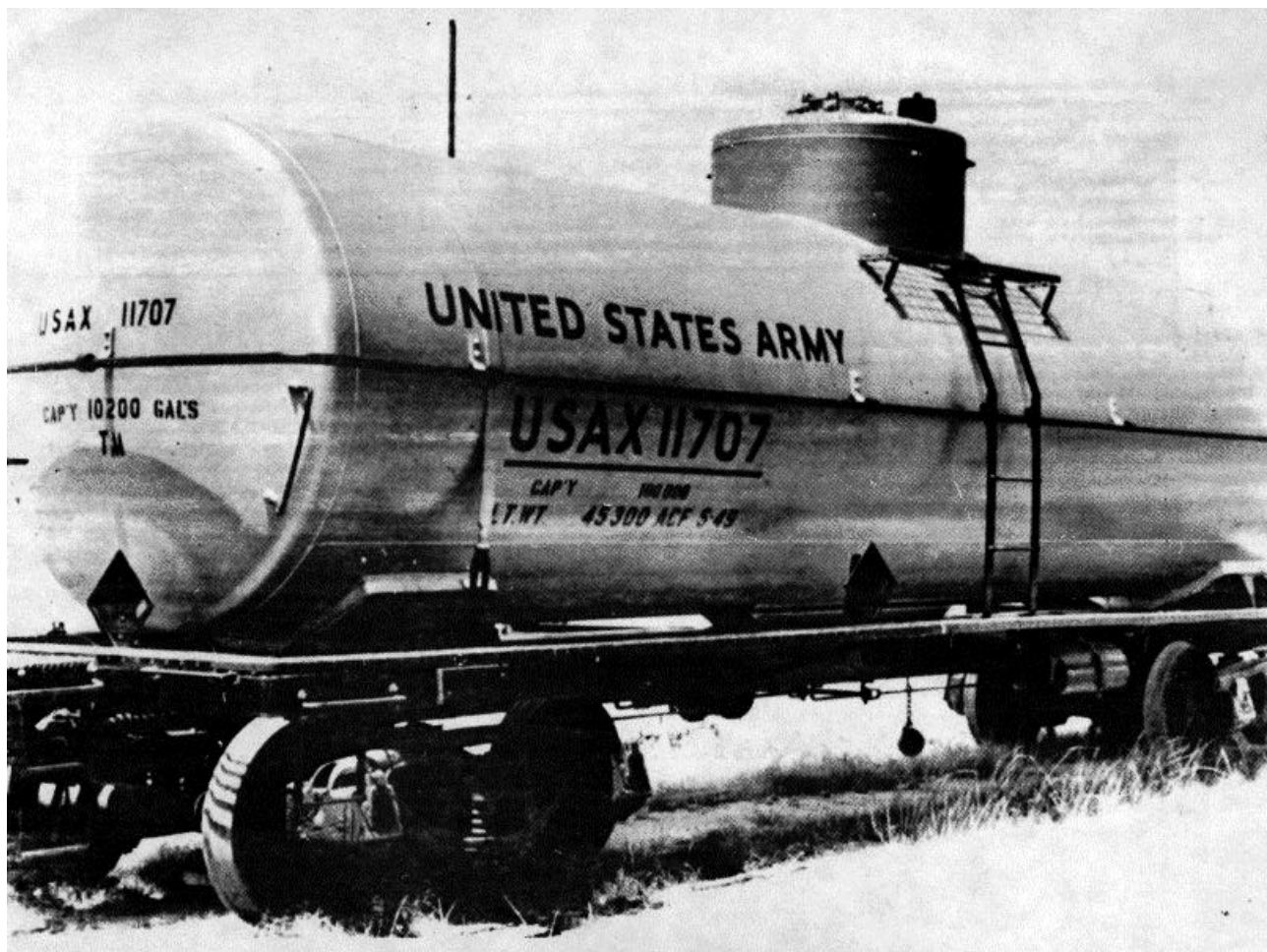
Figure 2-6. Railway tank car, petroleum, 56 ½-inch gage, 10,000-gallon 8-wheel, domestic service.
